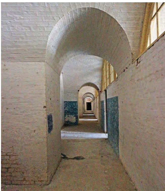
Interconnecting tunnel behind NE casemates
